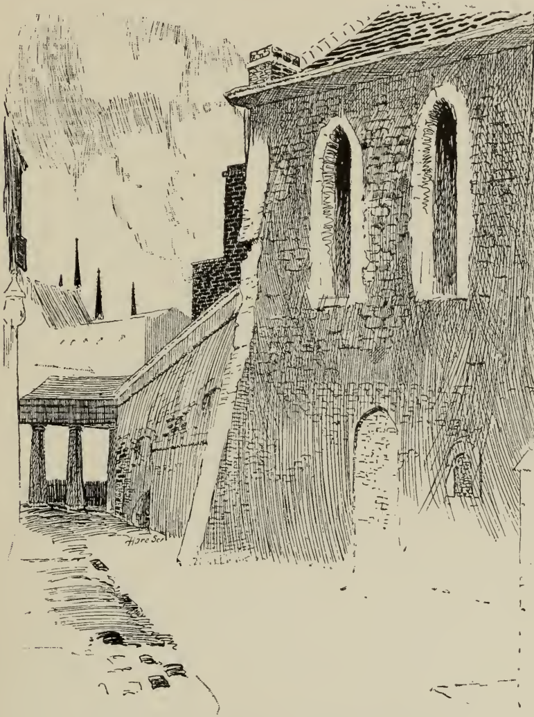
SOUTH SIDE OF THE PRINCE'S CHAMBER.
